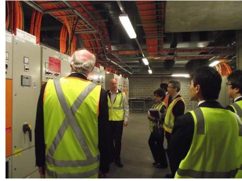
Lane Cove Tunnel 視察
